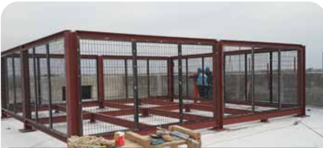
Platform ve Izgara İmalatı Platform and Grating Manufacturing
